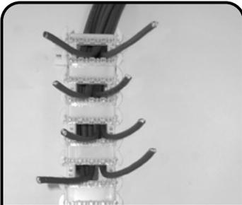
**3** Lace the cables through the appropriate openings in the wiring base and snap the S210™ wiring base onto the standoff bracket. Push the wiring base onto the stand-off bracket until the latches “snap” into place.
