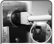
Insert the ZMAX Panel Jack into the back of the industrial outlet. Insure the key feature in the jack is oriented to match the key feature in the Industrial outlet.
