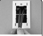
Pull cables through the appropriate openings in the faceplate and mount the faceplate to the electrical box with the screws provided.
