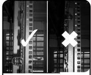
Locate the cable management fingers onto the frame rails as shown. NOTE: The fingers should be oriented so that the fingers point to the outside of the cabinet as shown.
